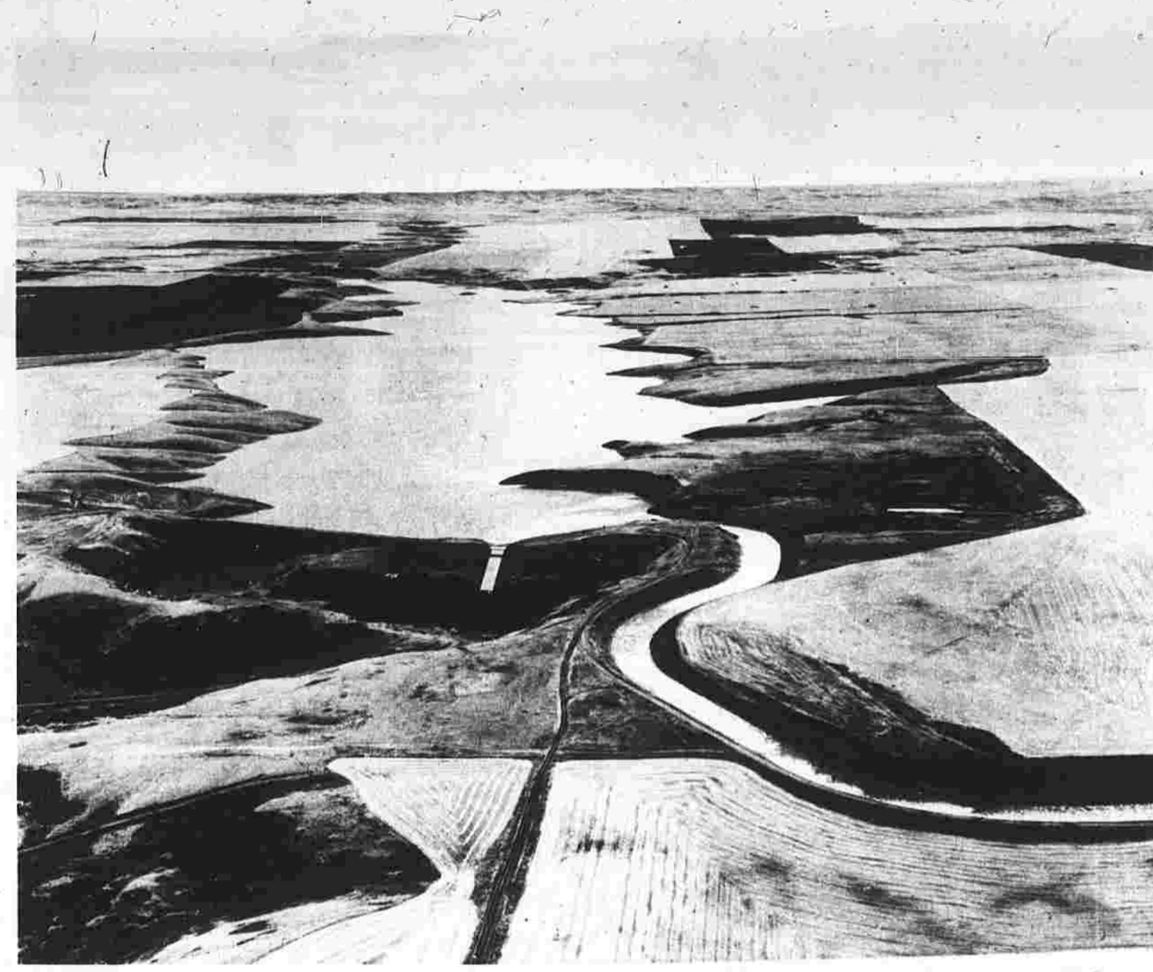
IRRIGATION DAM, WITH CANALS, IN SOUTHERN ALBERTA
